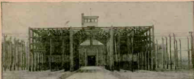
This "forest of switches" directs signals to any part of the world, from the new Voice of America.
